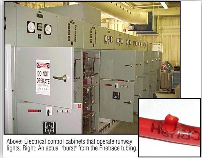
Above: Electrical control cabinets that operate runway lights. Right: An actual "burst" from the Firetrace tubing.
